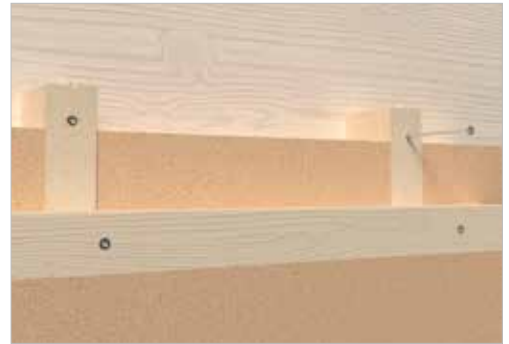
TTUFS screws in light wall framing.
